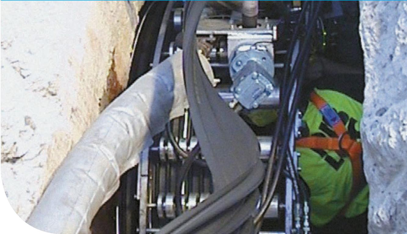
**A project in Sydney saw the unveiling of the next generation SEKISUI SPR spiral winding technology for structural lining of large diameter sewers.**
