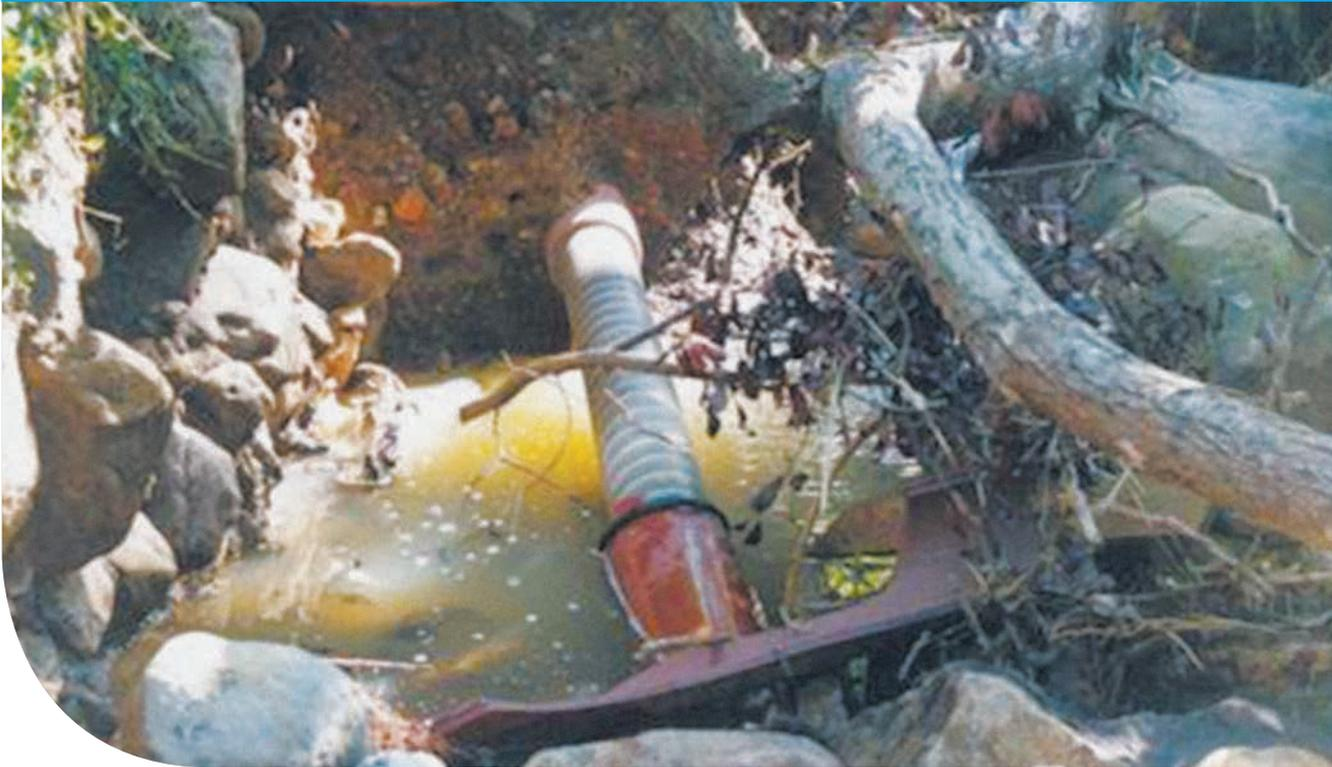
SPR™ EX liner intact inside the smashed vitrified clay pipe
