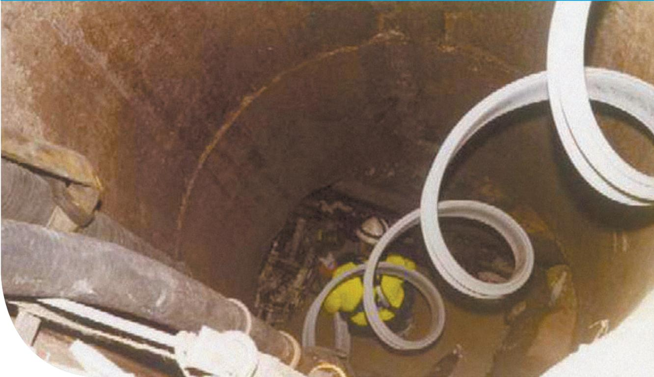
Rotaloc installation in a 6 metre (19.6 ft.) deep 1350mm (54 in.) diameter sewer in Geelong.
