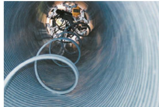
Winding of the SPR™ RO liner in the 160m (524 ft.) long pipeline was completed in a total of 4 working nights. External voids were filled with cementitious grout after this installation.
