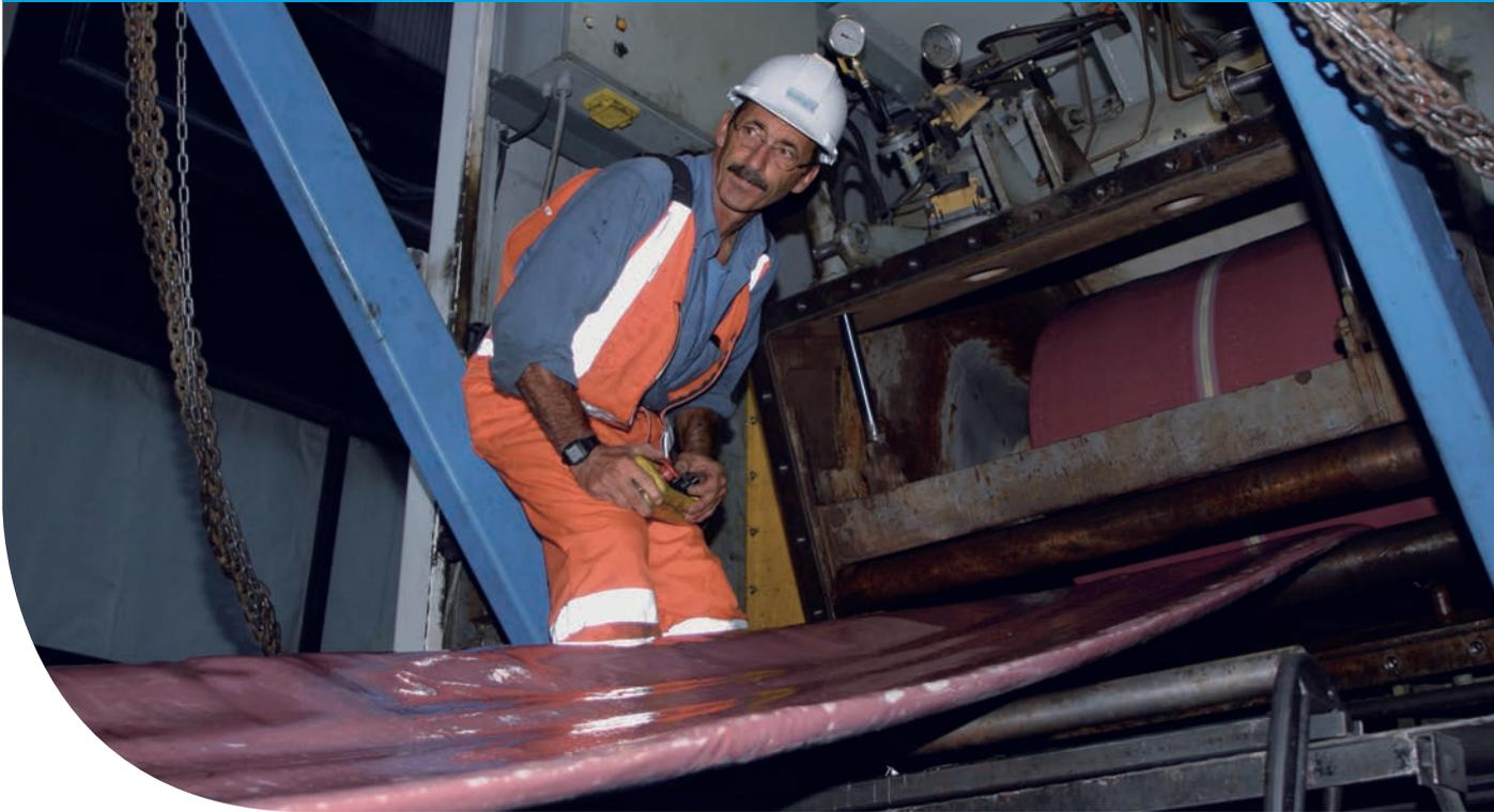
**The water pipes in the old section of Montreal, Canada, are over 100 years old. In a two-year project they are being effectively renewed with NORDIPIPE™.**
