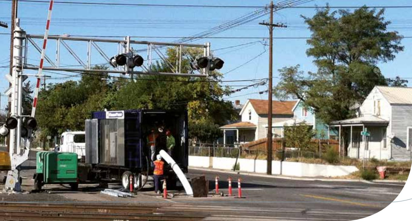
Installation of NORDIPIPE™ liner under six sets of Burlington-Northern railroad tracks.
