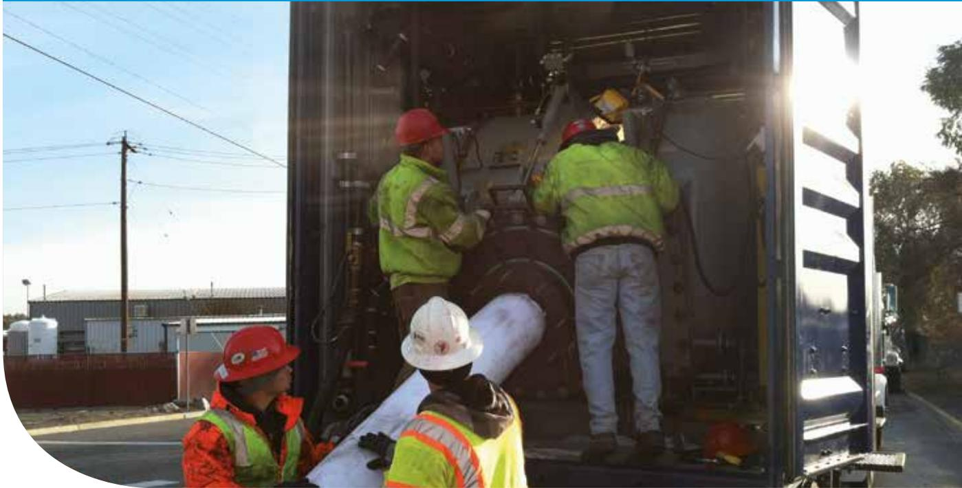
Installation of NORDIPIPE™ with pressure vessel.
