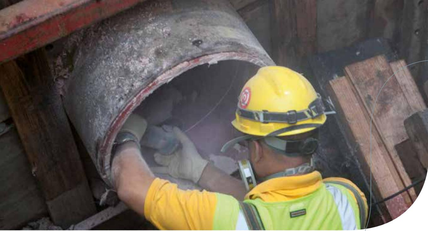
Here, a workman cuts off the end of the NORDIPIPE™. More than 500,000 feet of potable water lines in North America and Europe have been rehabilitated with NORDIPIPE™.
