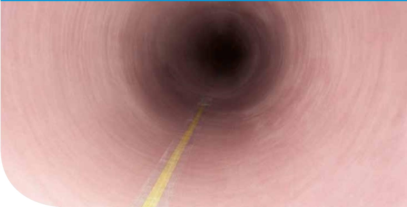
The 20-inch NORDIPIPE™ installed in Township of Montclair is jointless, NSF 61 certified and is designed for E80 loading. The service life is conservatively estimated at 50 years.
