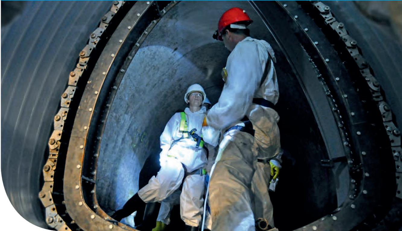
Rehabilitation with an interceptor beneath the Leuzetunnel. It was the largest diameter ever rehabilitated with the SPR™ Spiral-Wound in Germany.
