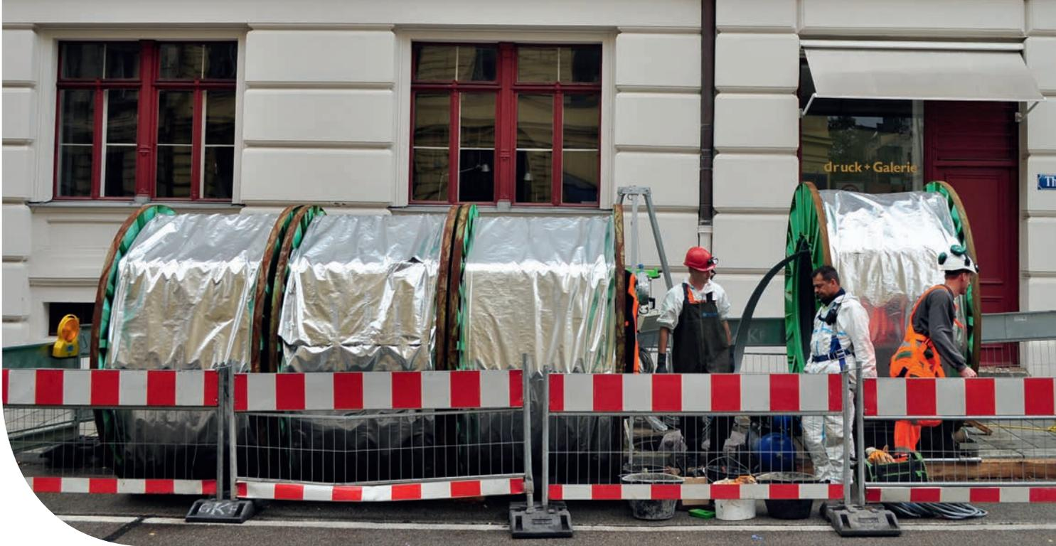
Before installing the spiral-wound pipe, KMG drained the rehabilitation sections and removed sinter deposits down to the core of the masonry, in order to expose the actual profile. Additionally, two data cables attached to the walls were moved elsewhere and protruding obstructions were milled off. The live flow from the adjoining properties was upheld by cutting open the liner promptly and sliding in a plastic pipe.
