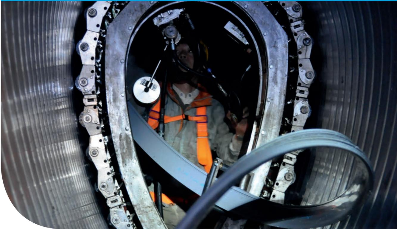
Pilot project for SPR™ technology during the rehabilitation of a combined sewer in Munich, Thierschstraße
